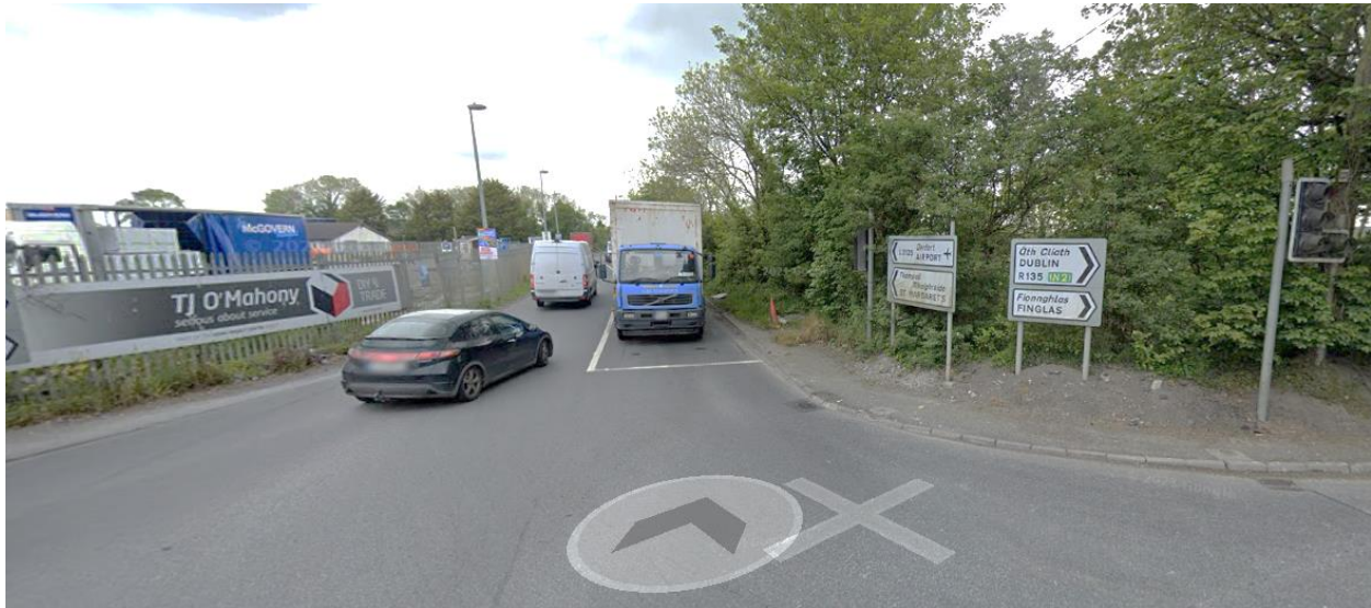
Figure 13a: Photo of L3125 arm on Kilshane Cross (Signalised) Junction (Adopted in EIAR for the Proposed RBSF Component in the 2018 Planning Application) (Source: Google Maps)
